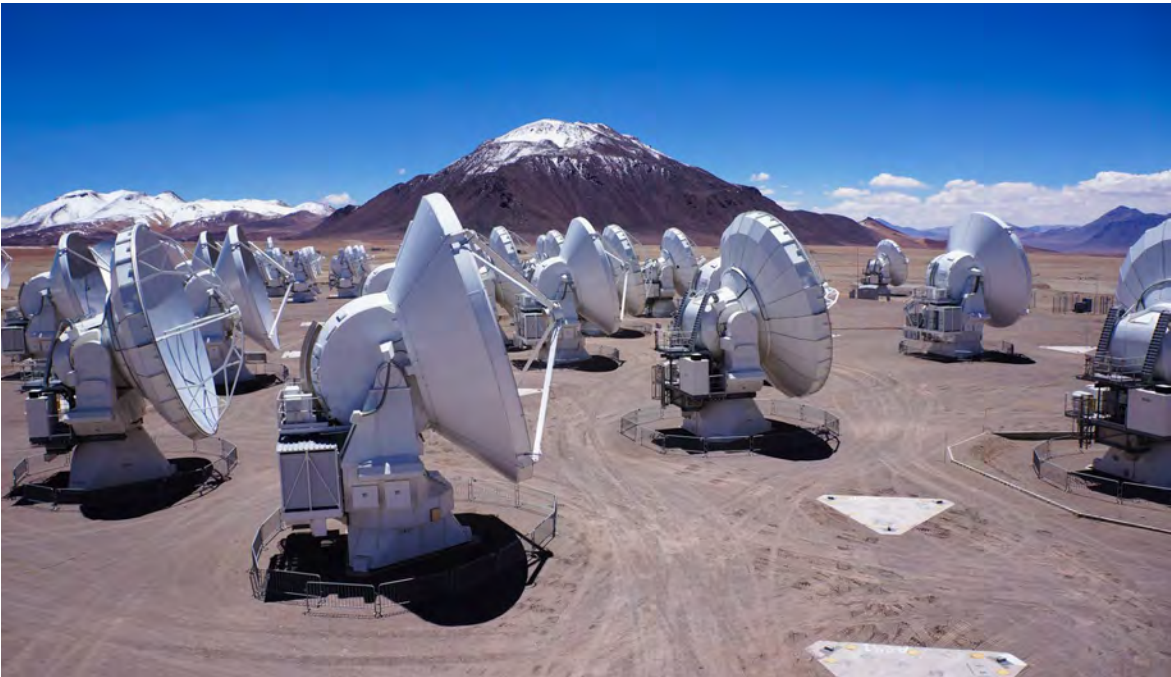
Figure 2.2: View of the inner core of the Atacama Large Millimeter/Submillimeter Array (ALMA) on the Chajnantor plateau (Chile) with the Cerro El Chascón (5703 m) in the background. A total of 66 antennas ( 12 \times 7 m diameter, 54 \times 12 m diameter) form the ALMA interferometer with baselines up to 16 km. The combined collecting area allows for high sensitivity while the interferometer setup provides unprecedented resolution in the submillimeter wavelengths. Credit: NRAO, P. Carillo
